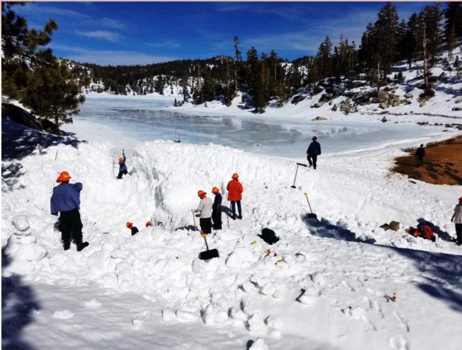
Emergency Spillway – March 14, 2017
