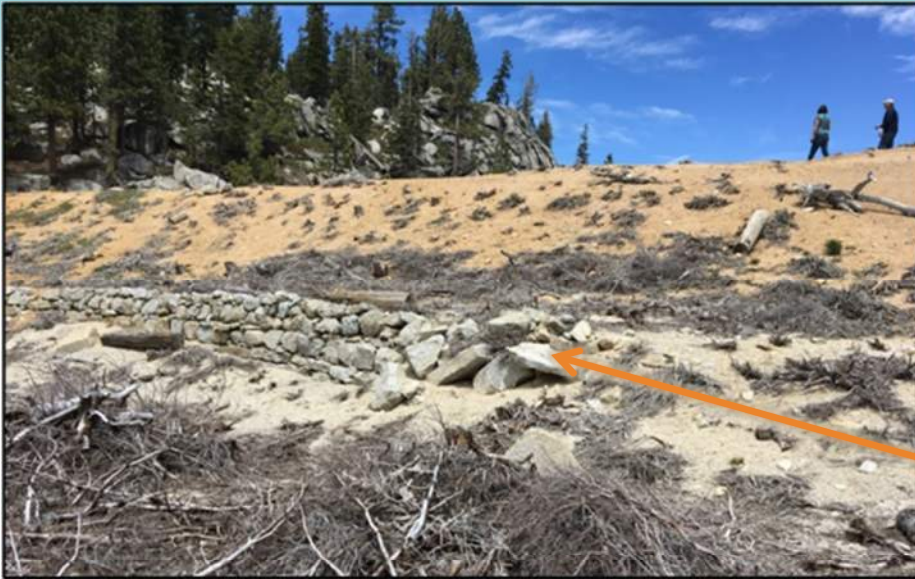
Existing Historic Wall
